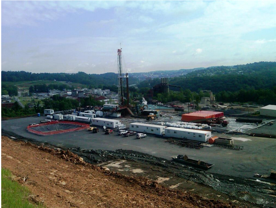
Figure 4. – MIP 4H drilling in June, 2011 showing the drilling operations on a state-of-the-art pad with berms and lining. The City of Morgantown is in the background.
